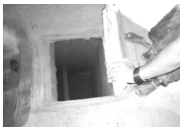
Fig 3. Kanagi storage bin
